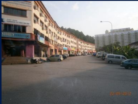
Rumah Kedai RK64 Taman Ukay Perdana 68000 Ampang Selangor 448 units Since 2009
