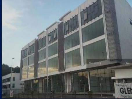
Glen 9 Hicom Glenmarie Shah Alam Selangor 24 units Since 2017
